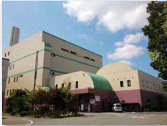
Ashiya City Refuse Disposal Center
